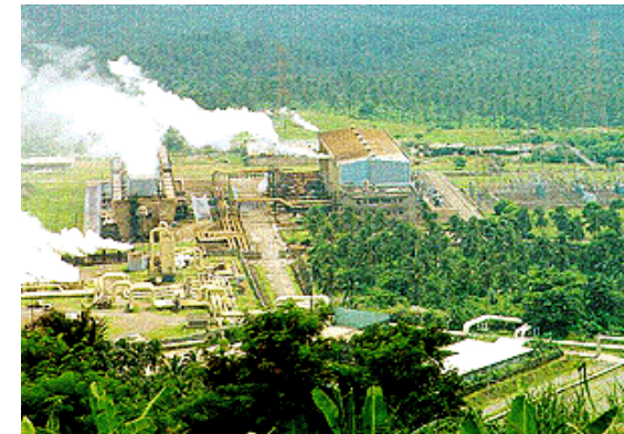
Makban Geothermal Power Plant Complex
