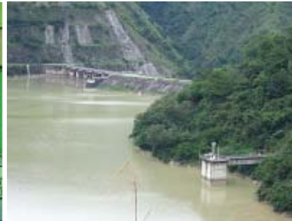
Binga Dam and Intake
