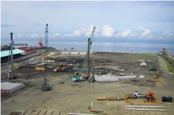
Ongoing Site Activities
