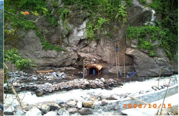
Tunnel B Inlet Portal
