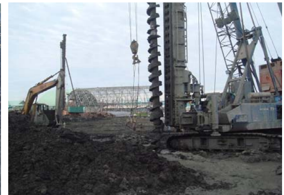
Pile work for TG
